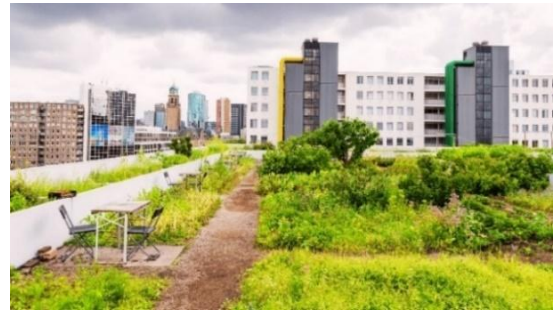
Figure 7: Intensive Green Roof
