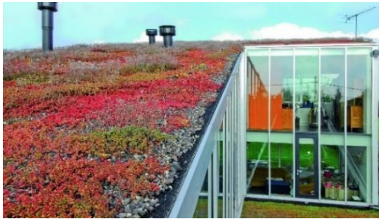
Figure 6: Extensive Green Roof
