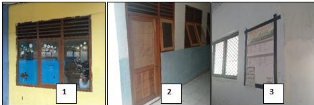
Figure 7. Condition of School Architecture and Furniture (1) Classroom windows of MTs Masyariqul Anwar which have not used trellises; (2) The design of the door of SDN Mekarjaya 3 which still opens inward; (3) Wall decorations that are pasted using masking tape instead of frames at SDN Tamanjaya 2.
