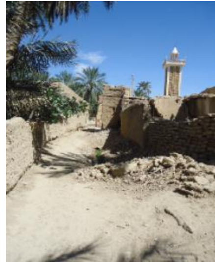
Fig 7. The deterioration of traditional buildings.
