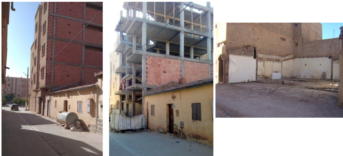
Figure 10.11.12 a traditional residence that was completely demolished and reconstruction with multiple floors by its owner ( Source: Authors. 2021. 2022)
