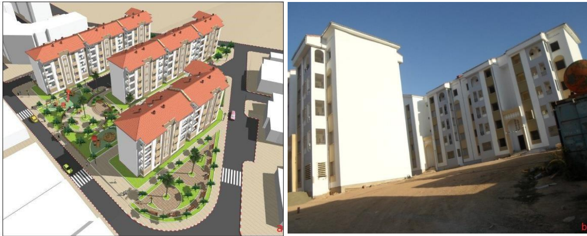
Figure 4: a, Views perspective of the HPE project [11]. b photo of the HPE project. Source author
