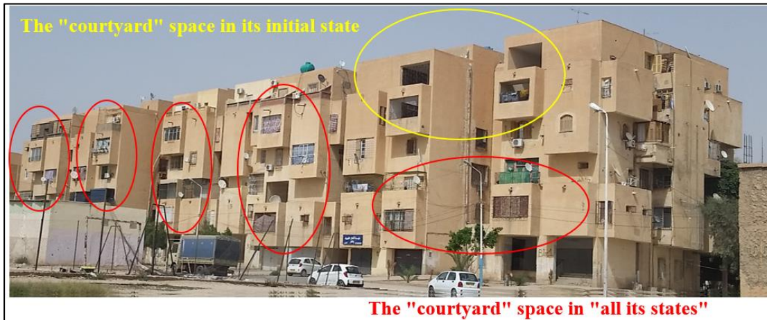
Figure 11. View showing the transformations of the city's facades by closing in different ways the open courtyards. (Source: author)
