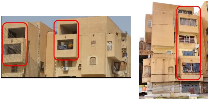
Figure 10. Left: the initial form of the courtyard Right: the various transformations of the courtyard (Source: author)
