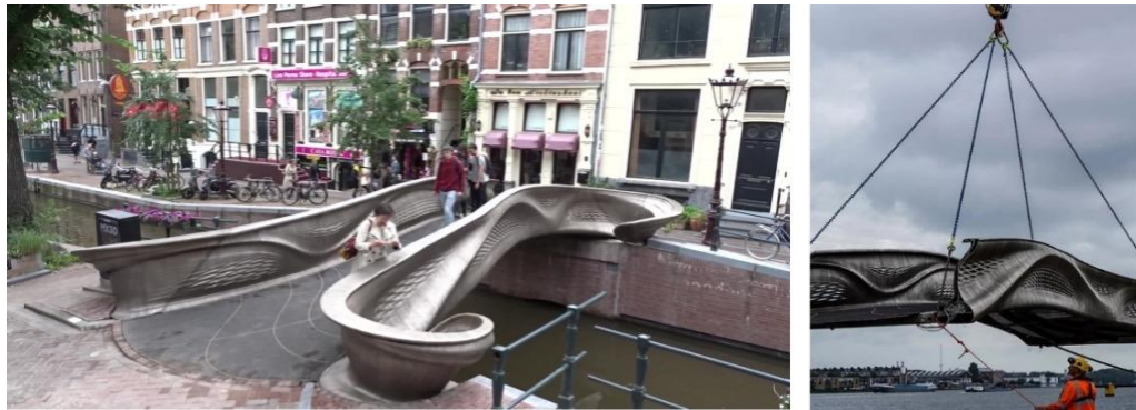
Figure 3. Smart Bridge Project in the Netherlands [23]
